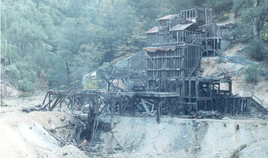
Afterthought Mine, Shasta County — Example of a Derelict Structure. (Photo courtesy of Phil Woodward, Central Valley Regional Water Quality Control Board)
